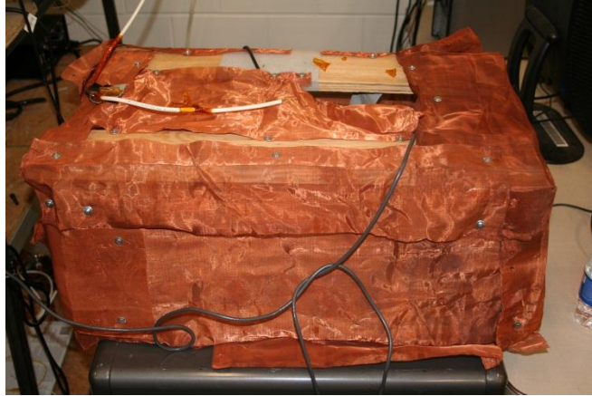
Figure B.3: The faraday cage is used to keep the high voltage transformer from picking up ambient noise.
