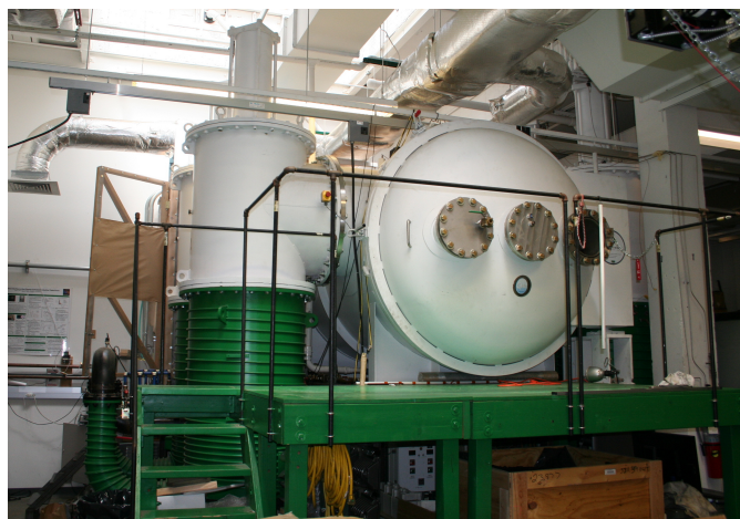
Figure 2.5. Large main chamber with diffusion pumps (seen in green) supporting MPX Mk.I. MPX quartz tube connected via a center port (18 inch diameter) at the rear.
